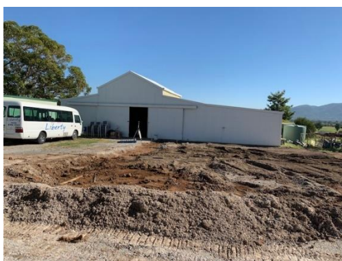
Site preparation for the new bus shed
